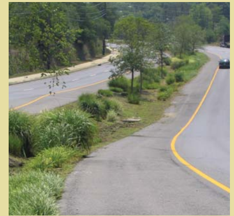
Low impact development median absorbs stormwater runoff from Adelphi Road in Prince George's County, Maryland.
